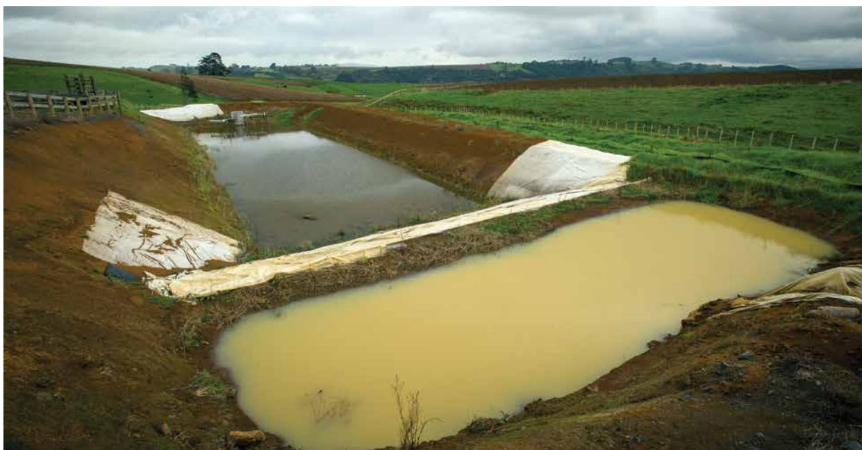
Sediment retention ponds meet NZGAP Environmental Management System (EMS) add-on best practice standards.
