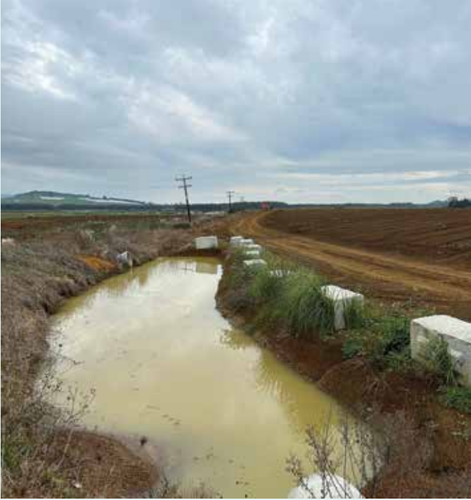
Effective sediment retention pond (silt trap) - Tuakau, Waikato (2024)
