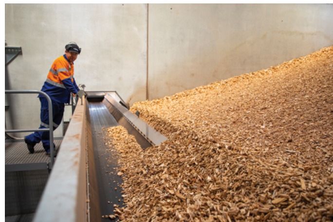
Wood chip in the storage facility moves onto the conveyer belt to be transported to the boiler
