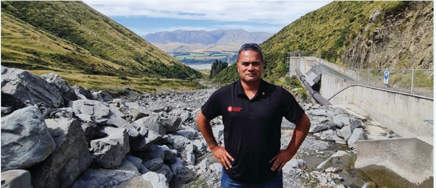
Anthony Taueki at the Clearwater Power Station intake in Canterbury
