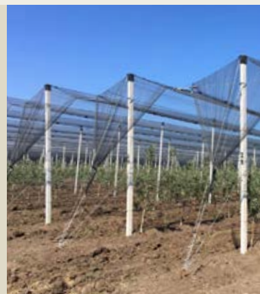
Concrete structure & Neutral Grey anti-hail net 10-12% shading
